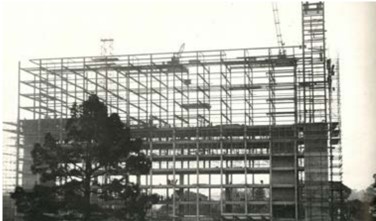
The welded steel frame in July 1960 (Melbourne School of Psychological Sciences archive)
